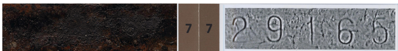
Corroded surface of plate
